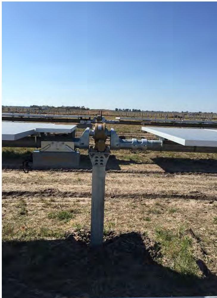
Plate 4: Indicative Single Axis Tracking
