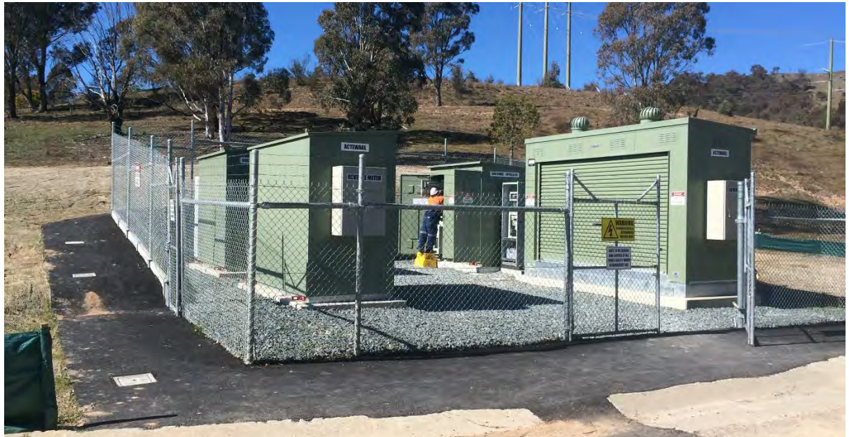
Plate 6: Typical Switching Station Arrangement
